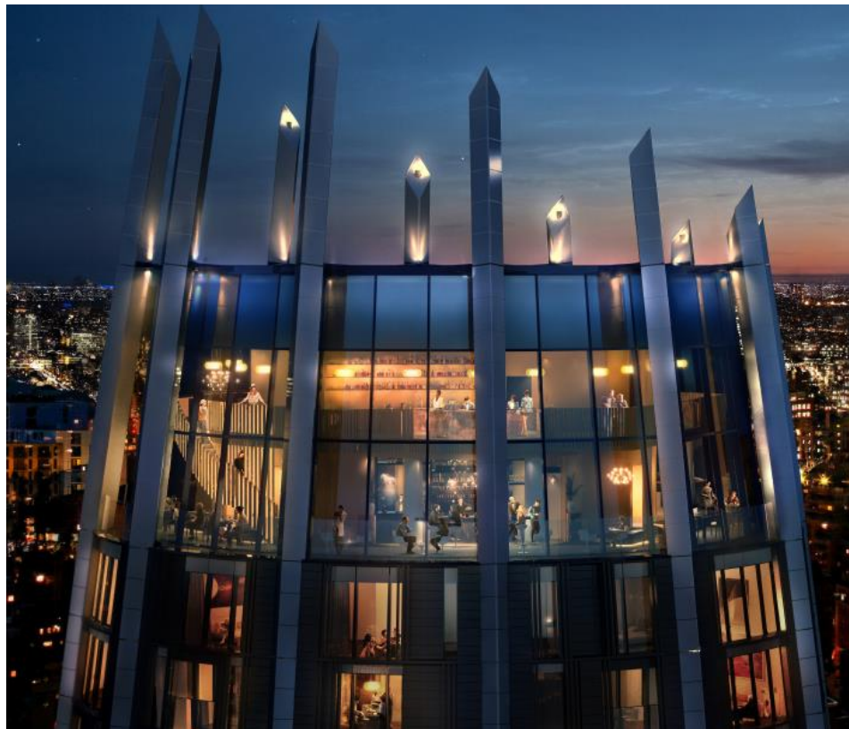
Detailed view of Building 1 façade (top) and view of top of building (sky bar over two floors) (bottom).
