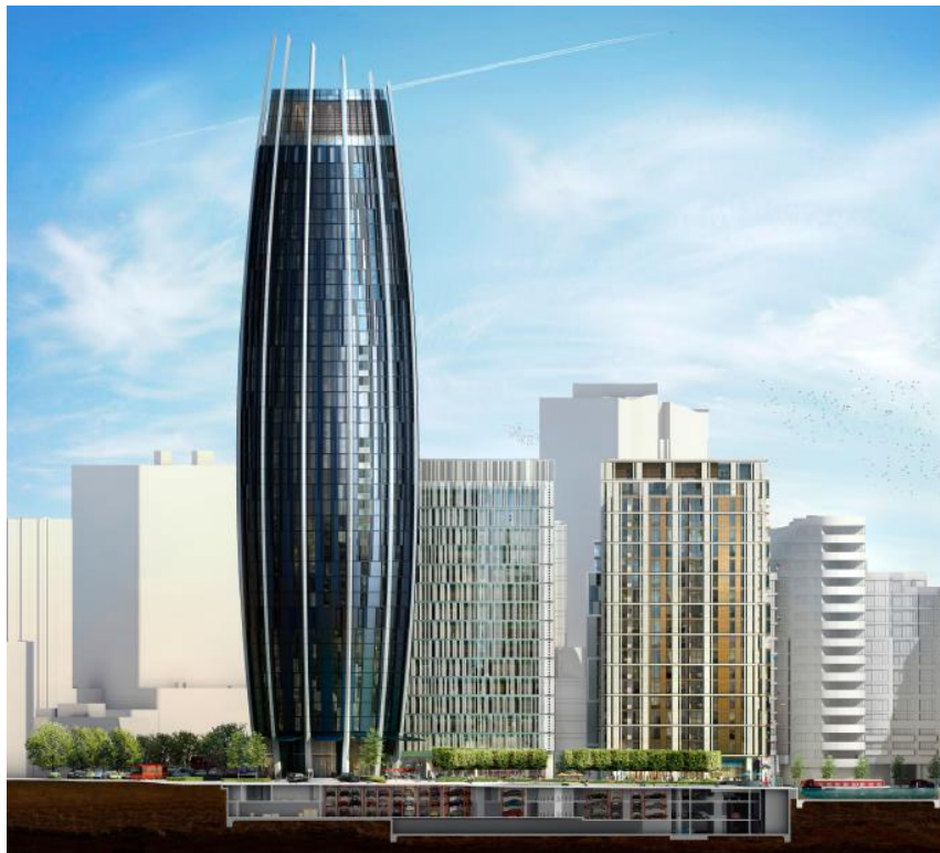
Aerial view of Merchant Square site showing Buildings 1 and 6 in context with surrounding buildings (top) and sectional view of Building 1 in context with Buildings 2 and 3 (bottom).
