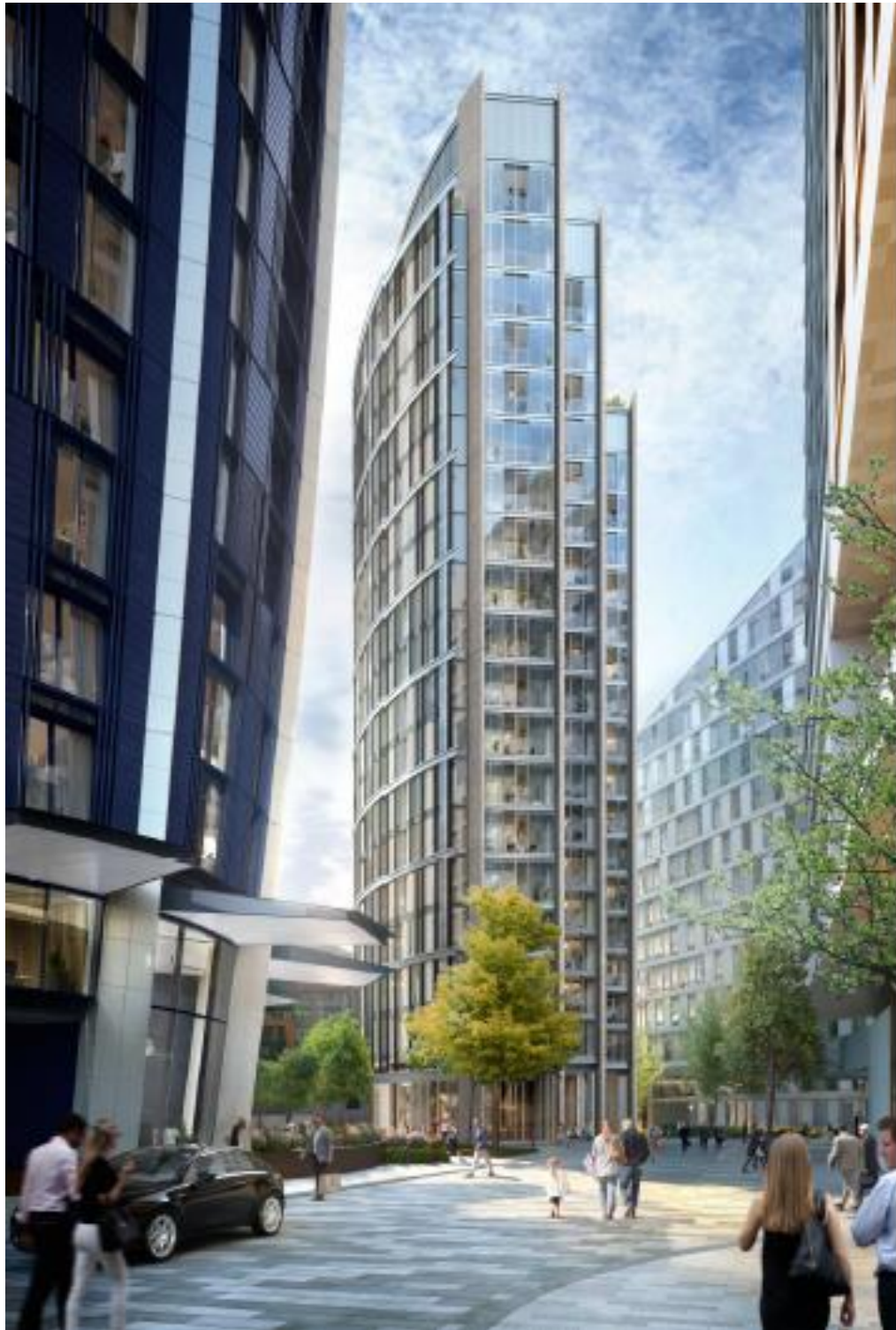
North elevation of Building 6 as seen from North Wharf Road.
