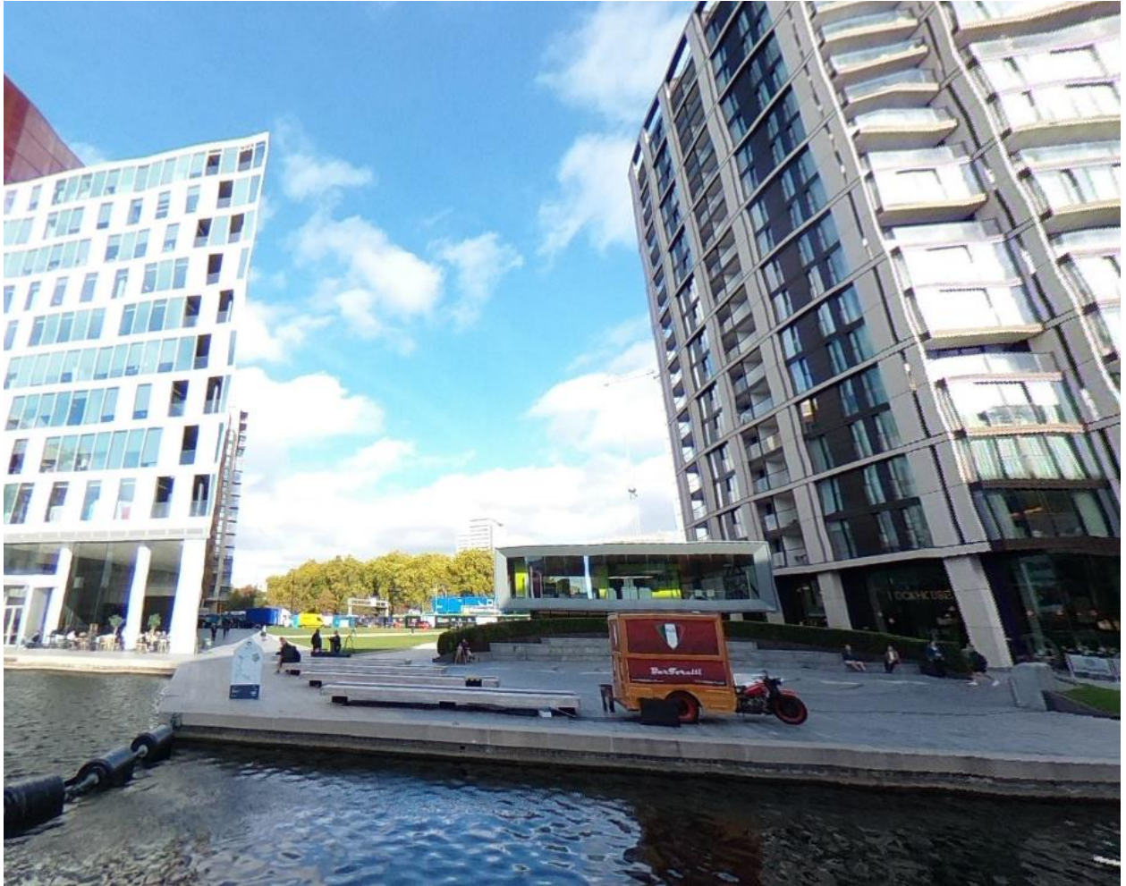
View of site from the south (site comprises land backward of the hard paved area in front of the two storey temporary marketing suite structure and between Building 5 on the left and Building 3 on the right).
