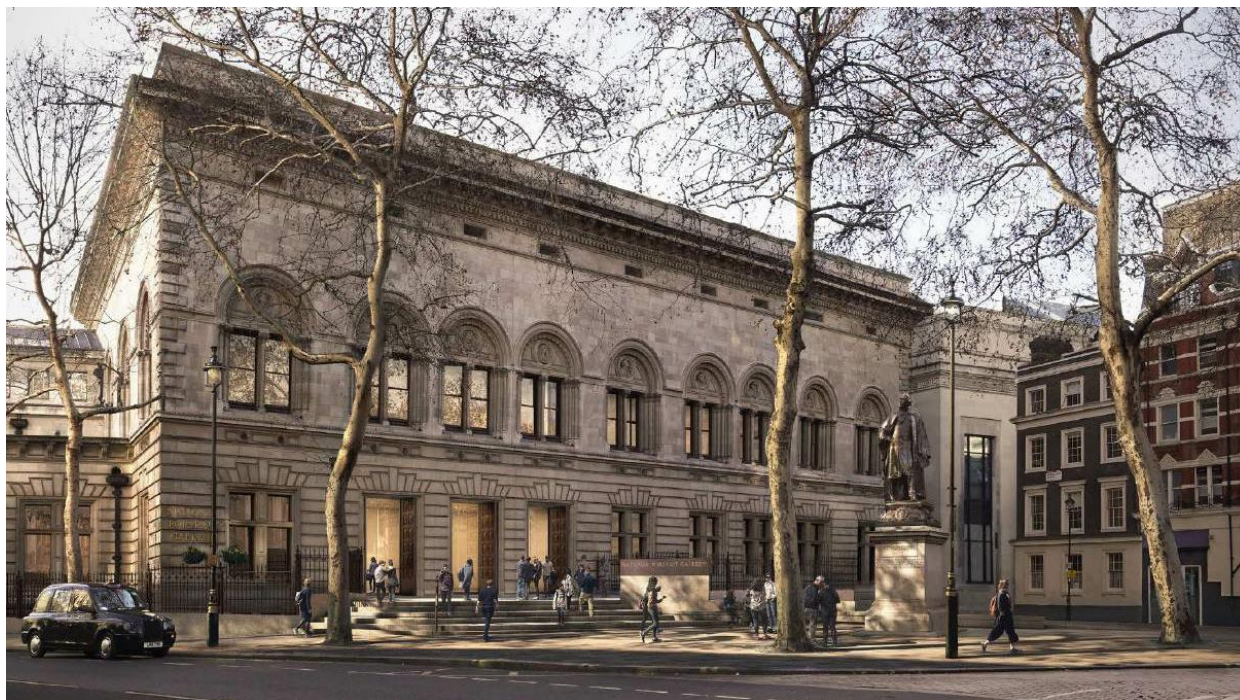
Computer Generated Image of Northern Façade
